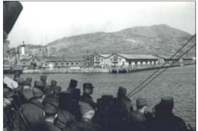
Cold morning at the Port of Pusan
